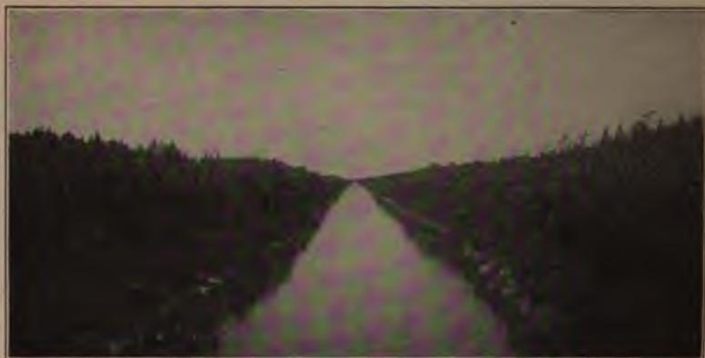
Drainage Ditch excavated by Floating Dipper Dredge.
